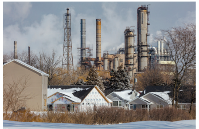
Matthew Kaplan, Whiting Refinery , photograph
